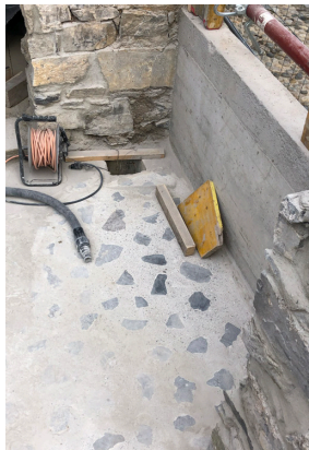
▲ Grinding of the Terrazzo floor.
