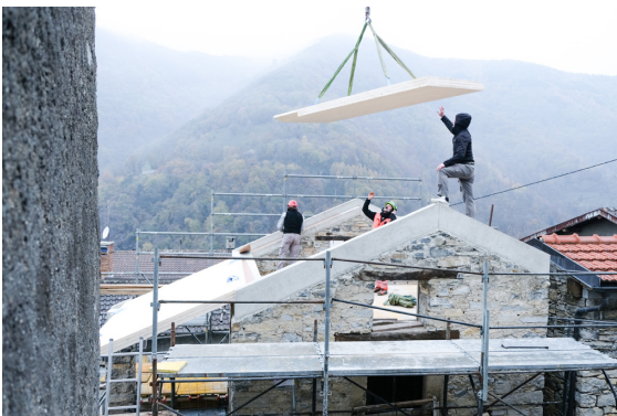
▲ Helicopter installation of the new roof structure. The detail of the new support was designed to allow for a thin roof overhang.
