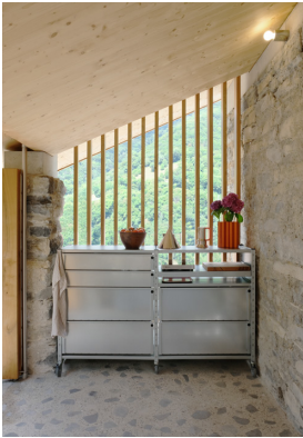
▲ Reuse of old chestnut wood and stone remnants for the kitchen's pavement.
